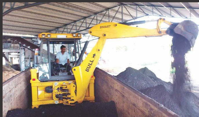
Backhoe Unloading Inside Truck
